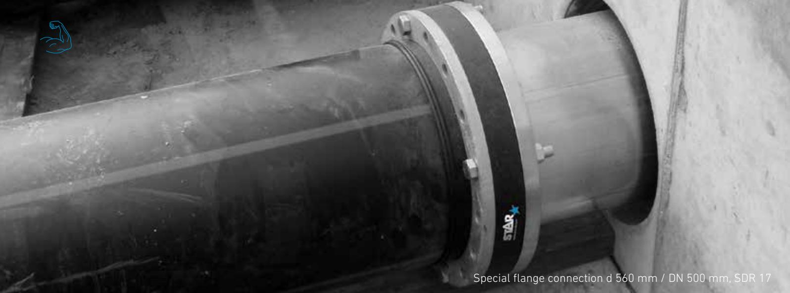
Special flange connection d 560 mm / DN 500 mm, SDR 17
